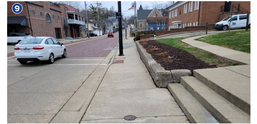
On the street next to the Armory building, the sidewalks narrow slightly. Amenities such as lighting and decorative poles exist throughout this segment. Still, as shown in the picture above, they are sometimes placed in a way that narrows the sidewalk further and can limit accessibility.
