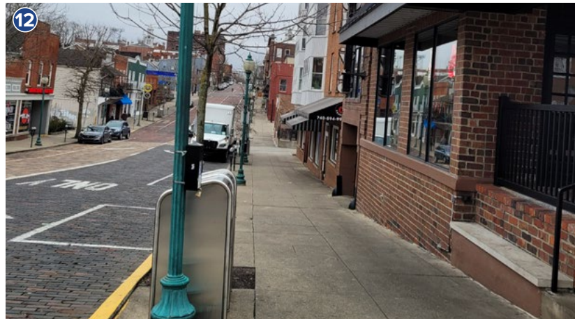
Looking south from the intersection of Court Street and Stimson Avenue shows a wide sidewalk ornamented with street trees, banners, street lights, and other decorative features. A sidewalk of this width encourages pedestrian activity, creating an attractive and inviting street life. Enough space exists on this sidewalk to facilitate high pedestrian traffic.
