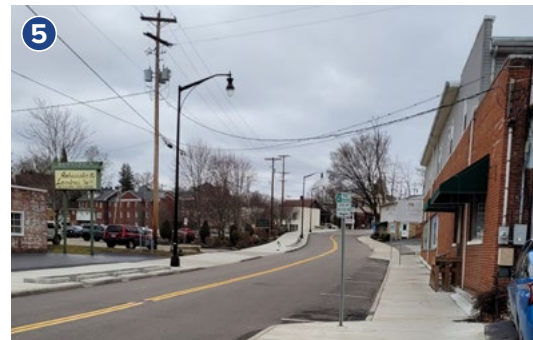
Multiple curb cuts intersect sidewalks along this area of Stimson Avenue, which could cause dangers for pedestrians. The sidewalks in this area also appear slightly wider than in the previous images.
