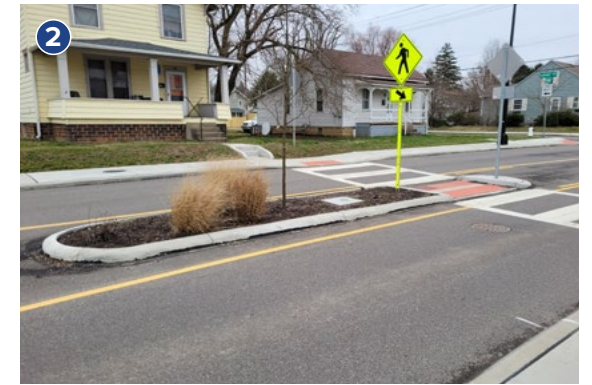
Sidewalks are in good condition along the eastern segment of mostly residential housing. However, no buffer is provided between the sidewalk and the street. A crosswalk with a pedestrian island allows for safe crossings, as seen in the image above.
