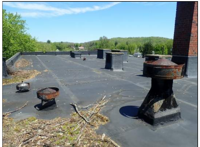
Overview of roof
