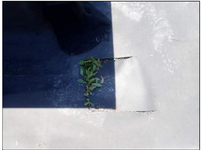
Cut-in membrane roofing
