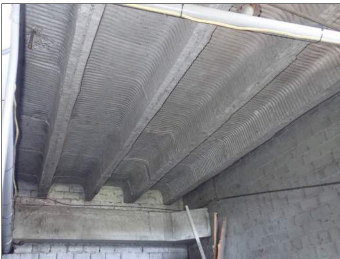
Typical second-story floor slab of northern section
