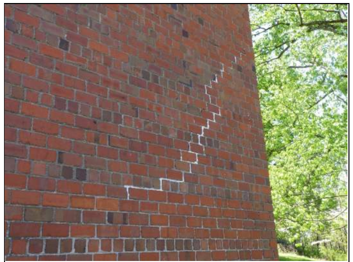
Typical sealant over mortar
