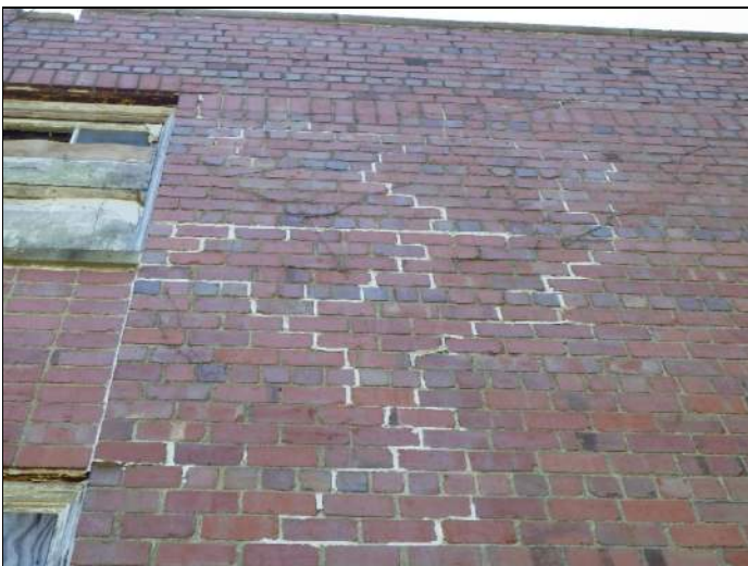
Typical sealant over mortar
