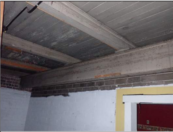
Typical roof framing of southern section
