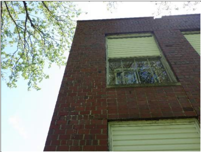
Typical wood-framed window
