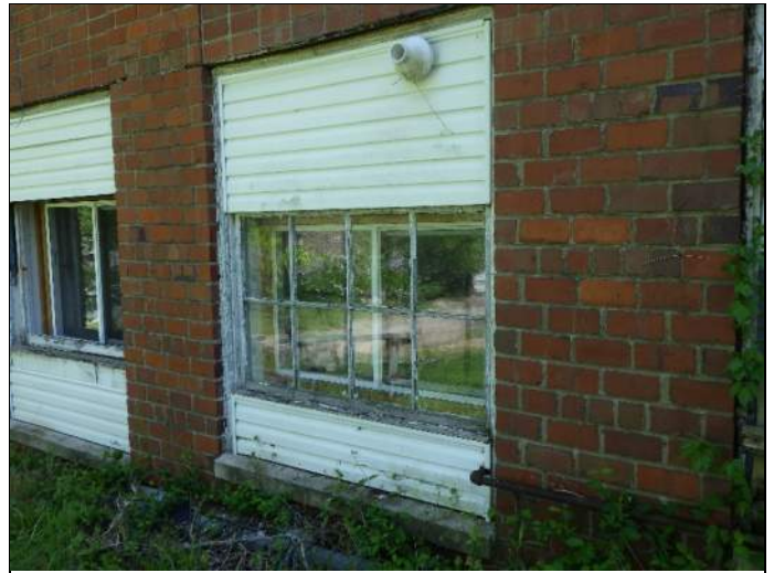
Typical wood-framed window
