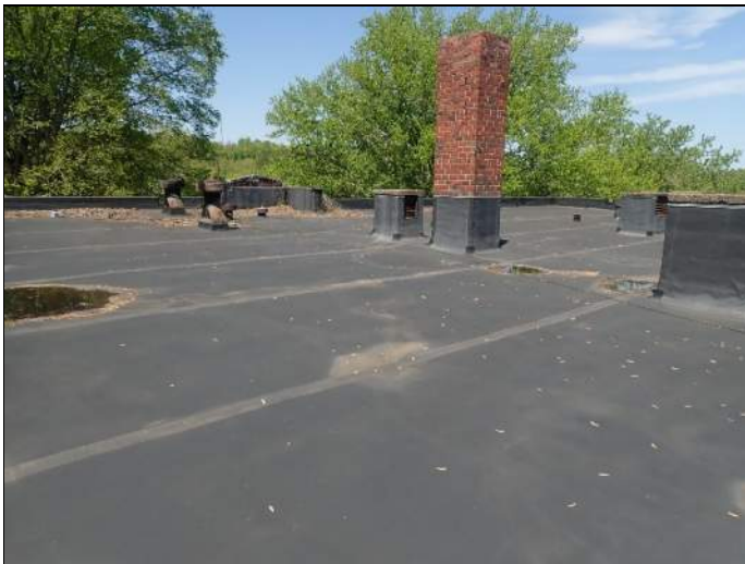
Overview of roof
