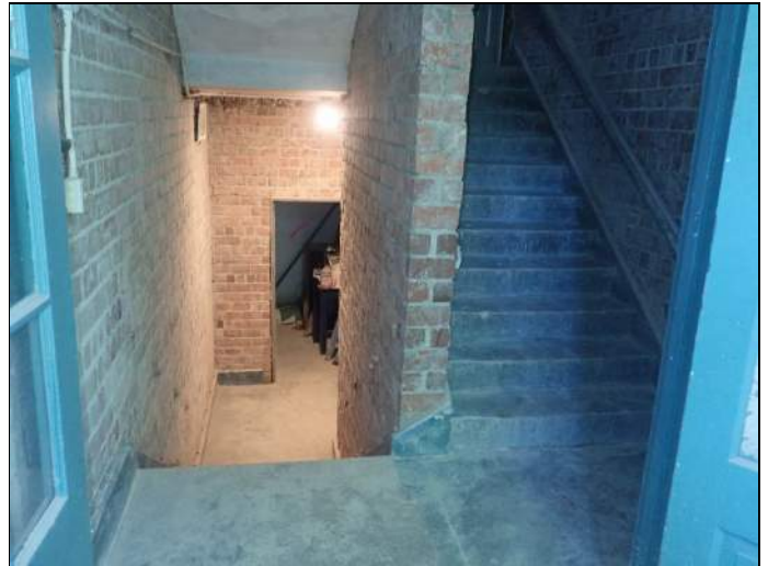
Stairs at front entrance
