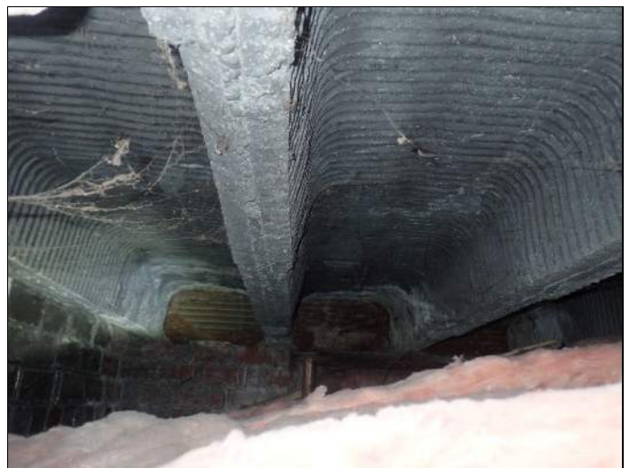
Typical second-story floor slab of northern section
