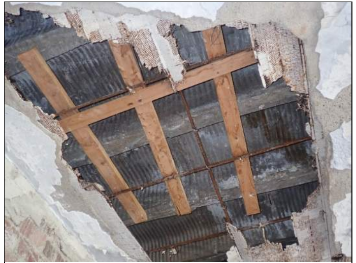
Typical roof slab of northern section
