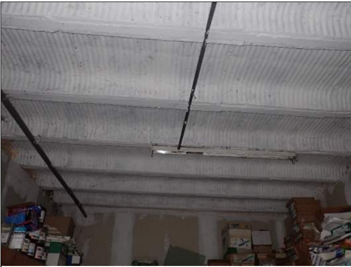
Typical second-story floor slab of northern section
