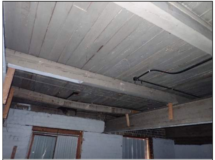
Typical roof framing of southern section
