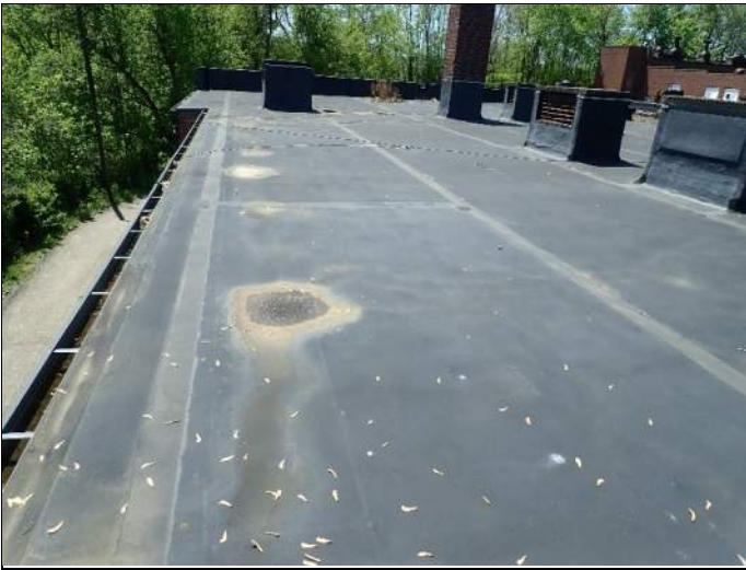
Gutter along east roof edge
