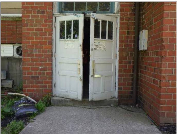
Typical wooden door
