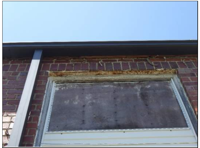
Gutter and downspout
