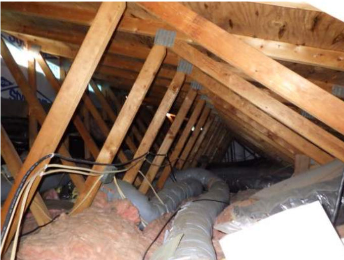
Overview of roof structure of east building
