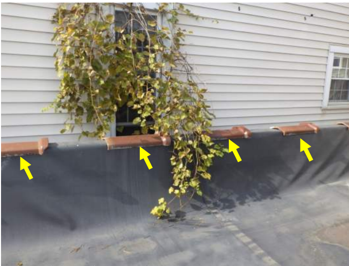
Clay coping tiles along west parapet
