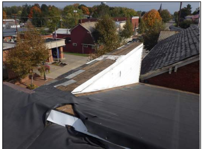
Overview of roof, looking east
