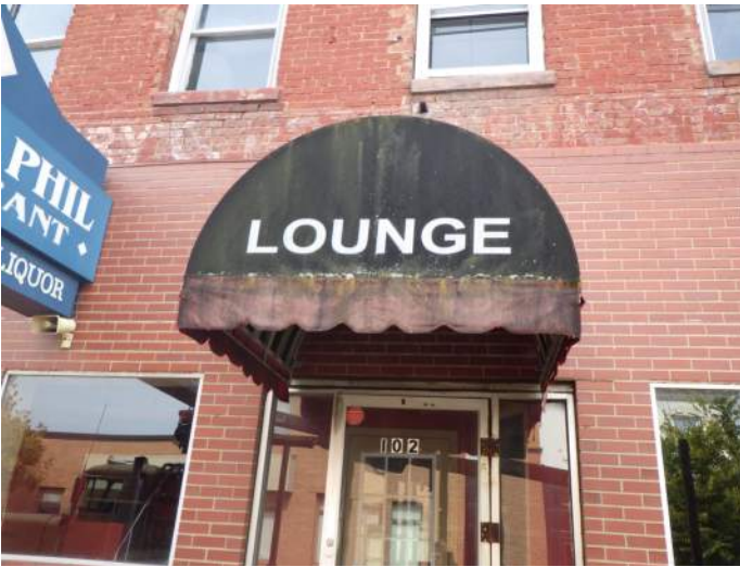
Typical entrance canopy
