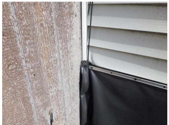
Termination bar along vinyl siding
