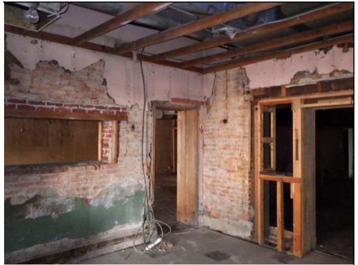
Overview of first story of west building
