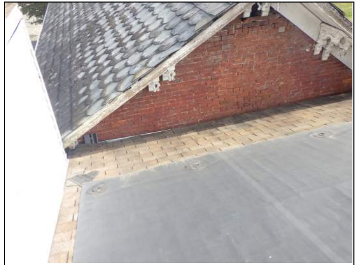
Roof edge against adjacent building
