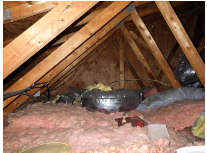
Overview of roof structure of east building
