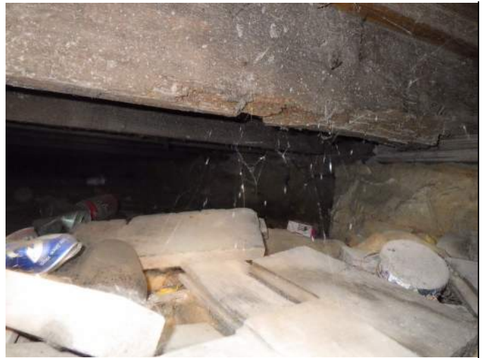
Overview of crawlspace
