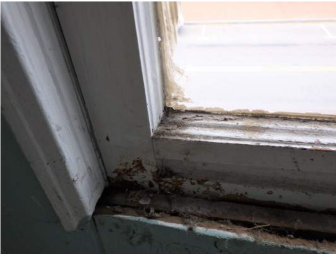
Typical window condition
