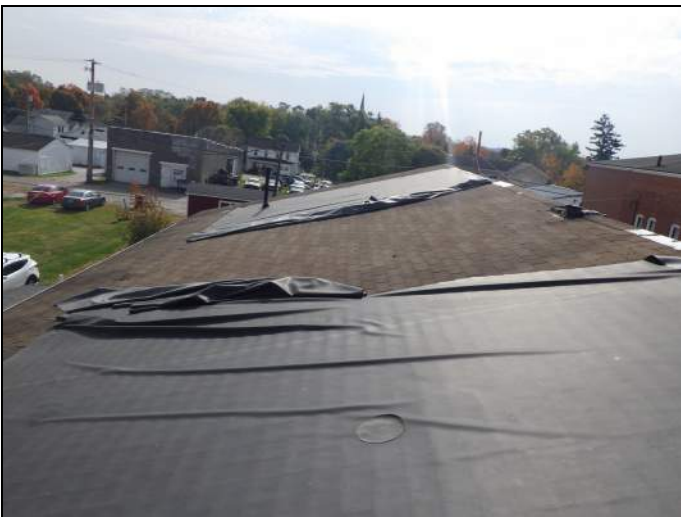
Overview of roof, looking south
