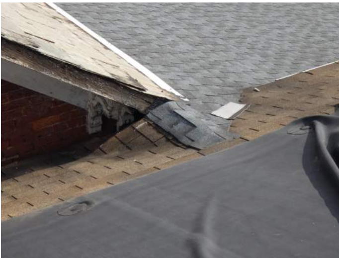
Roof edge against adjacent building
