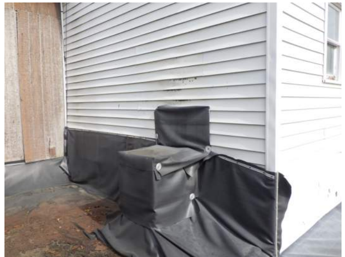
Termination bar along vinyl siding
