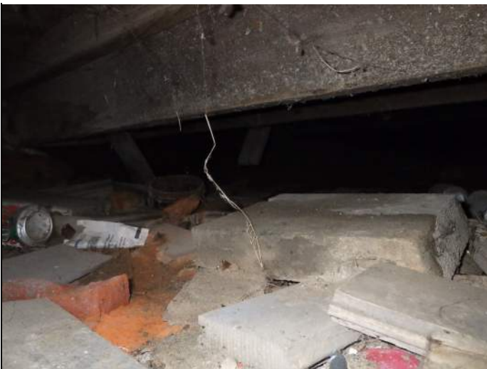
Overview of crawlspace
