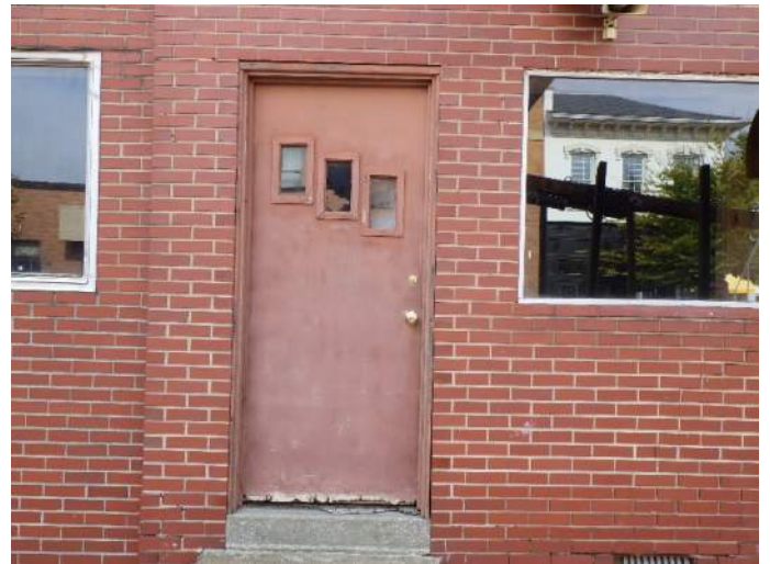
Wood door to second-story
