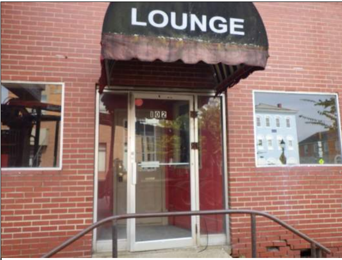
Aluminum-framed storefront system
