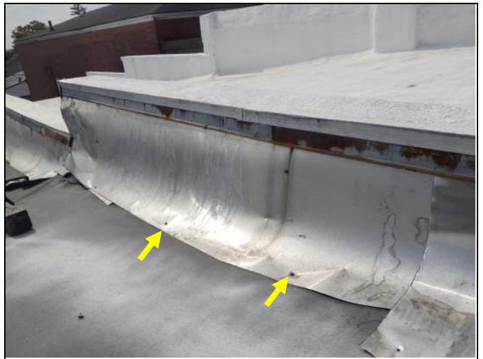
Sheet metal flashing, note screw fasteners
