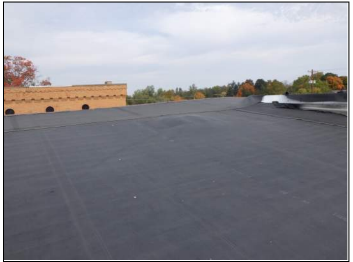
Overview of upper roof looking north
