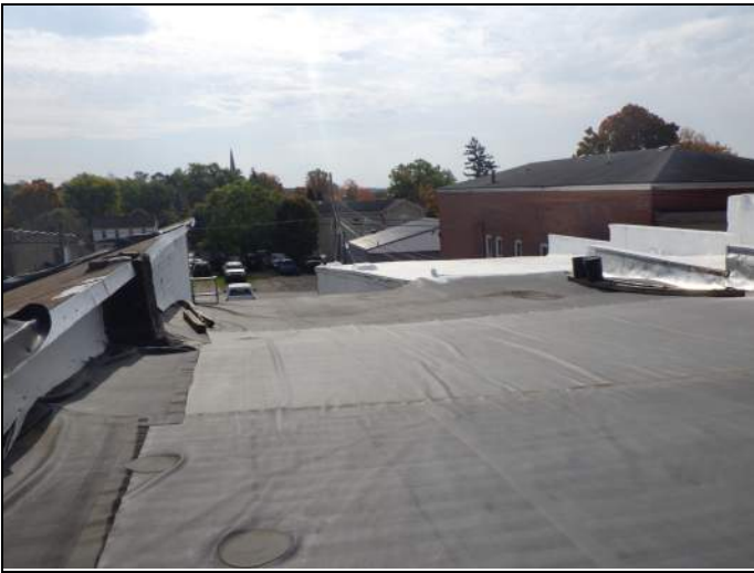
Overview of upper roof looking south
