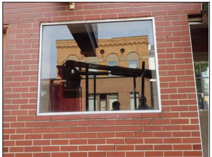
Single-pane metal-frame window
