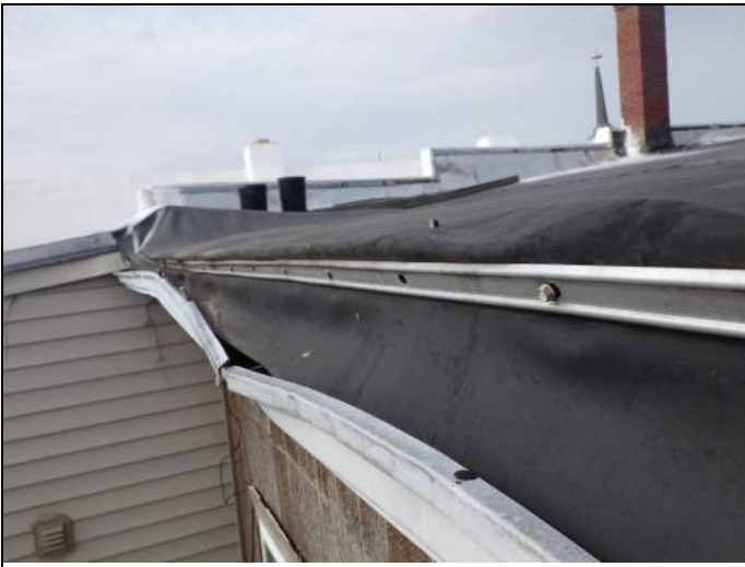
Gutter along south roof edge
