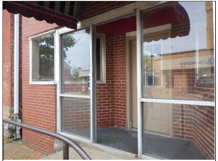
Aluminum-framed storefront system
