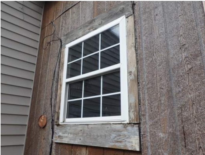
Typical vinyl-frame window
