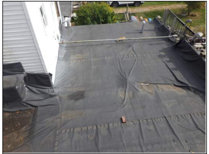
Overview of lower roof
