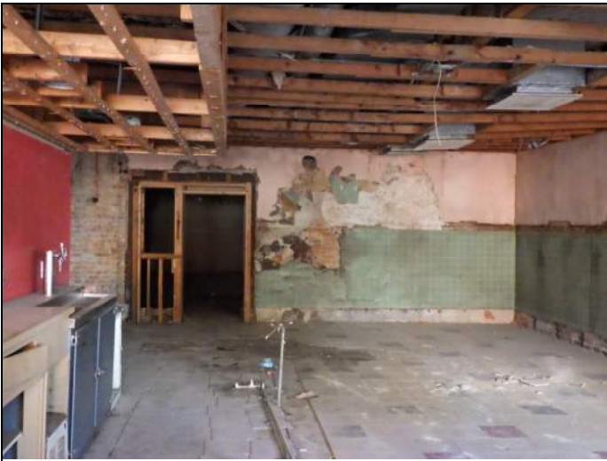
Overview of first story of west building
