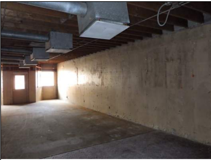
Overview of first story of east building
