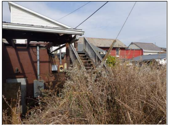
Stairs to first story at rear
