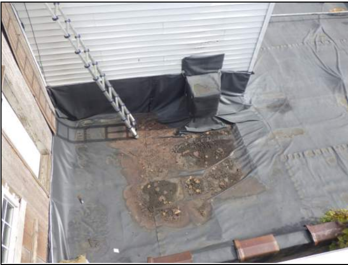
Overview of lower roof
