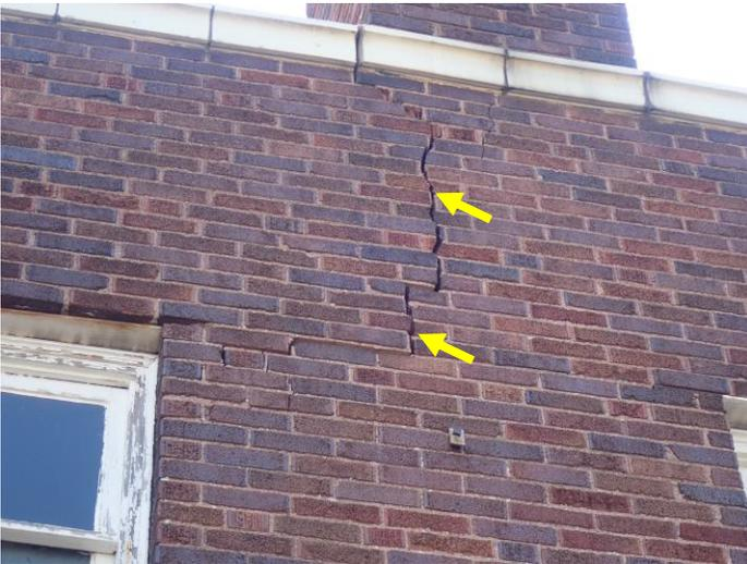
Cracked brick masonry at corroded lintel
