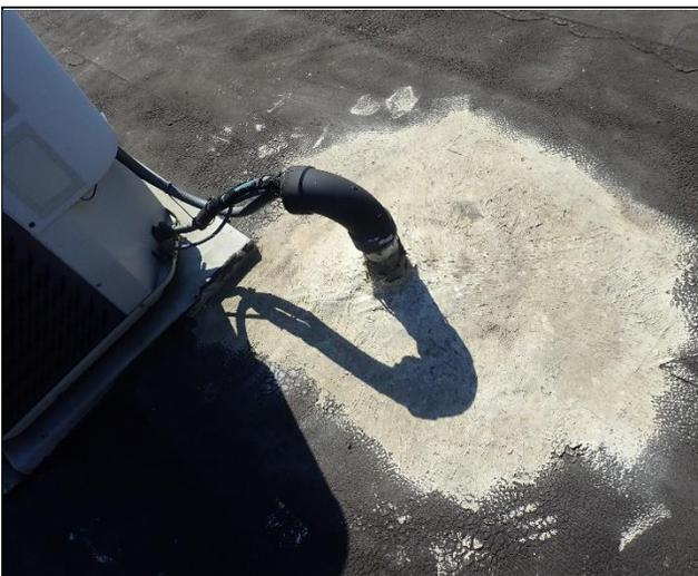
Deteriorated sealant at roof penetration
