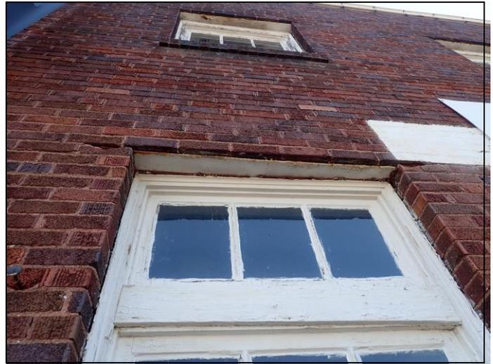
Corroded and expanded lintel
