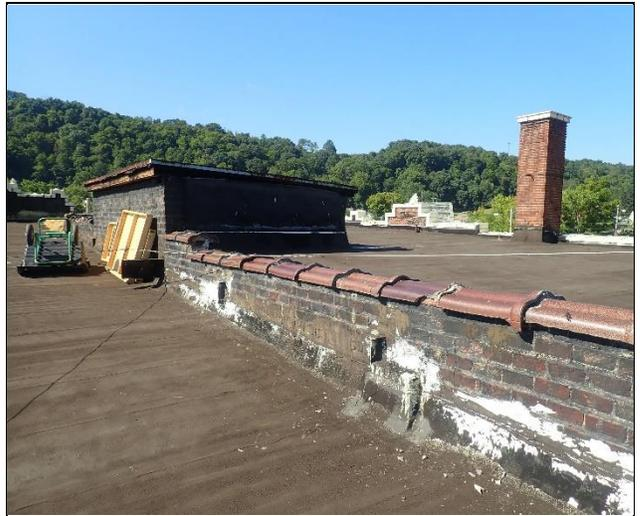
Cracked coping tile and deteriorated sealant
