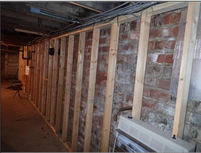
Typical supplemental wood wall framing in basement
