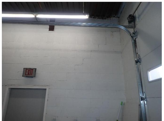
Stair-step cracking in exterior CMU wall
