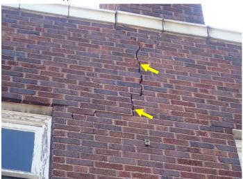
Cracked brick masonry at corroded lintel
