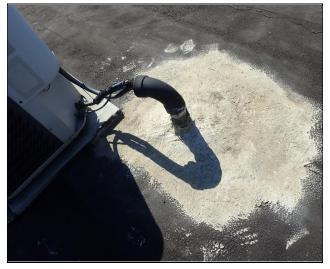
Deteriorated sealant at roof penetration
