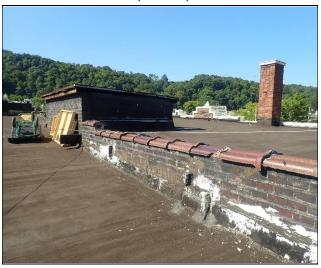
Cracked coping tile and deteriorated sealant
