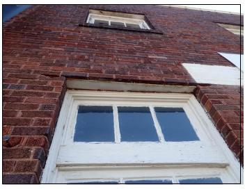
Corroded and expanded lintel
