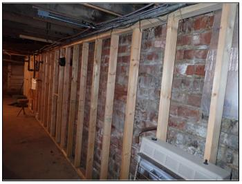
Typical supplemental wood wall framing in basement
