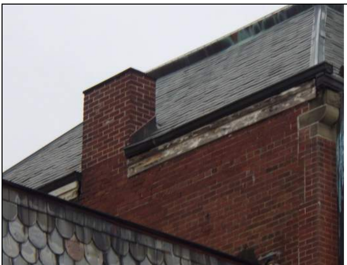
Overview of main building roof
