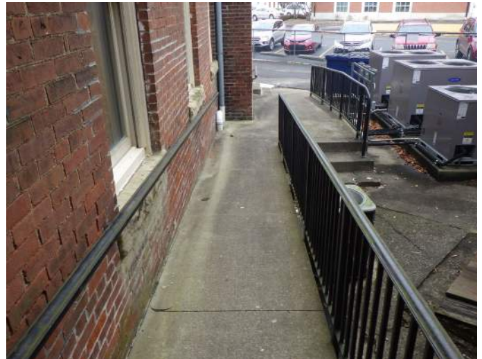
Accessible ramp in alley to auditorium
