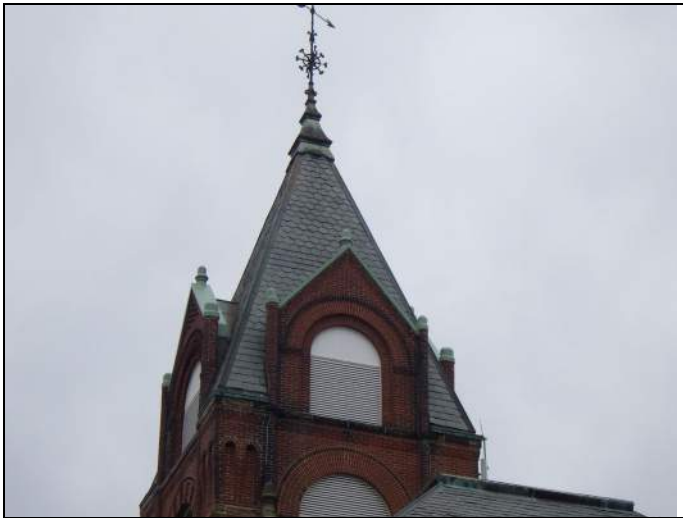
Overview of tower roof
