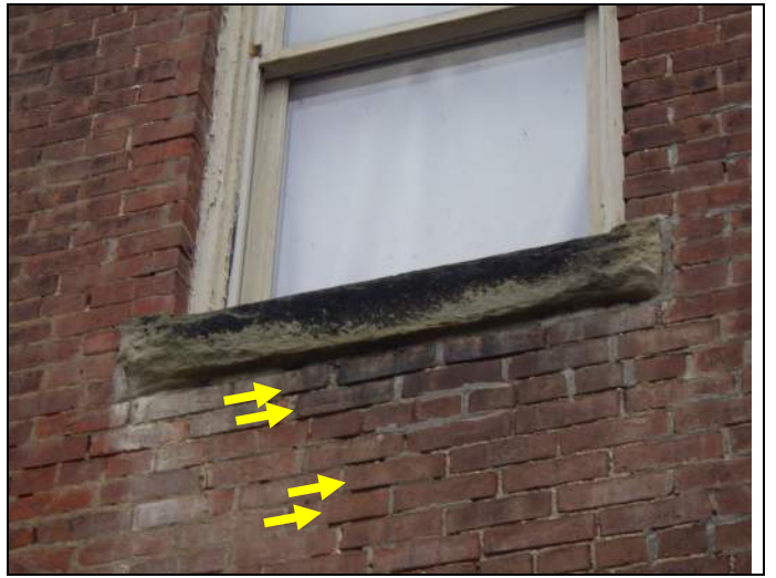
Deteriorated mortar
