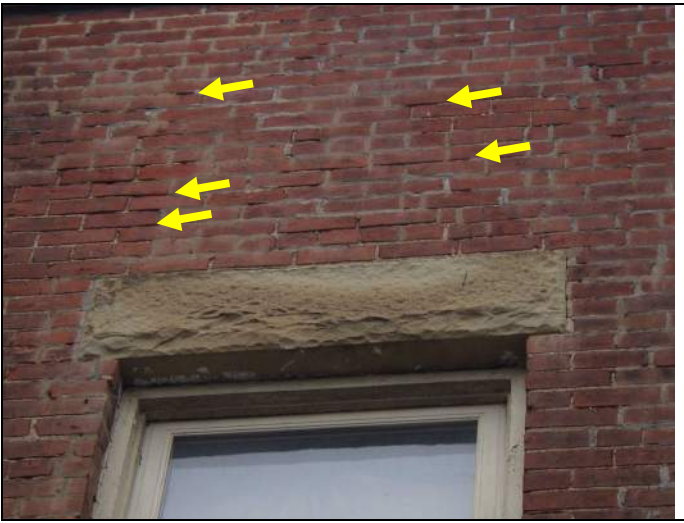
Deteriorated mortar
