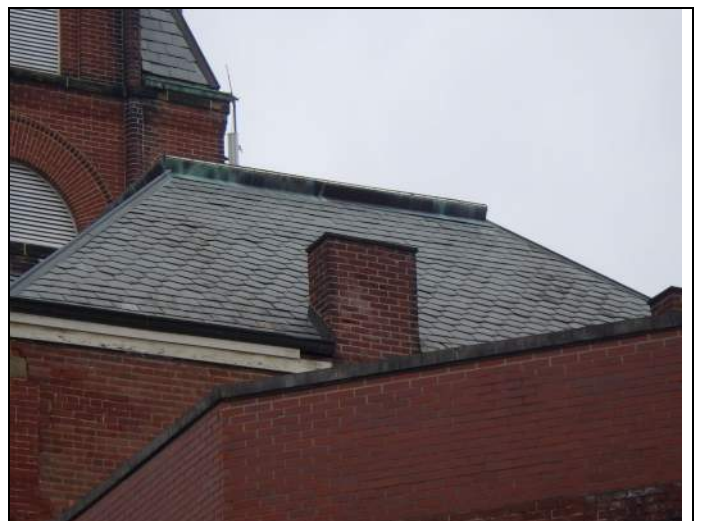
Overview of main building roof
