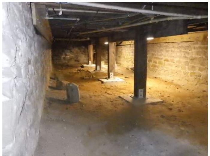
Overview of basement
