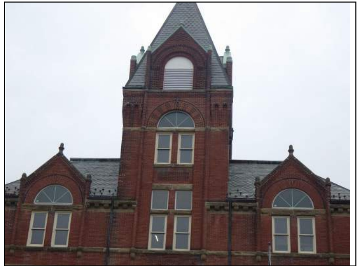
Overview of main building roof
