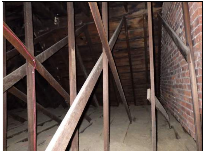
Overview of roof framing
