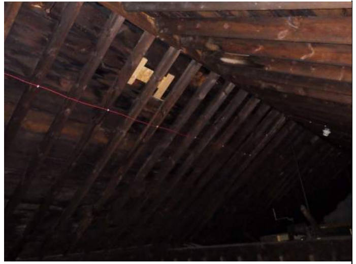
Overview of roof framing
