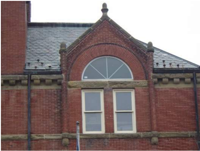
Typical vinyl windows
