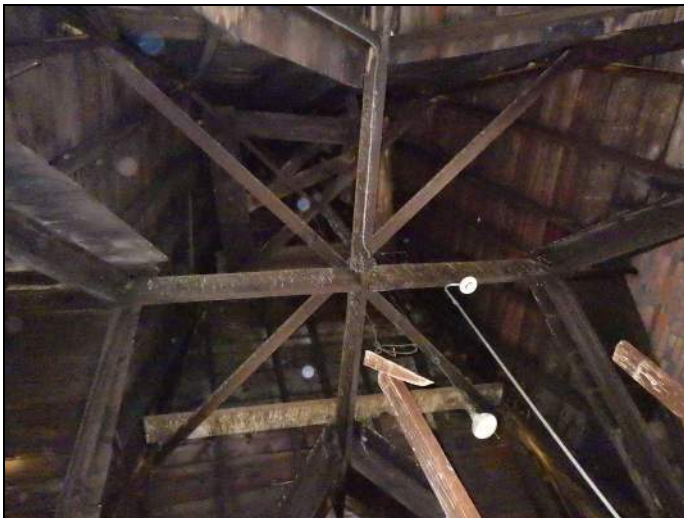
Wood-framed roof framing of tower
