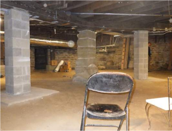
Water stains along valley rafter
