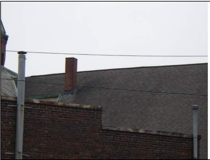
Overview of shingled roof
