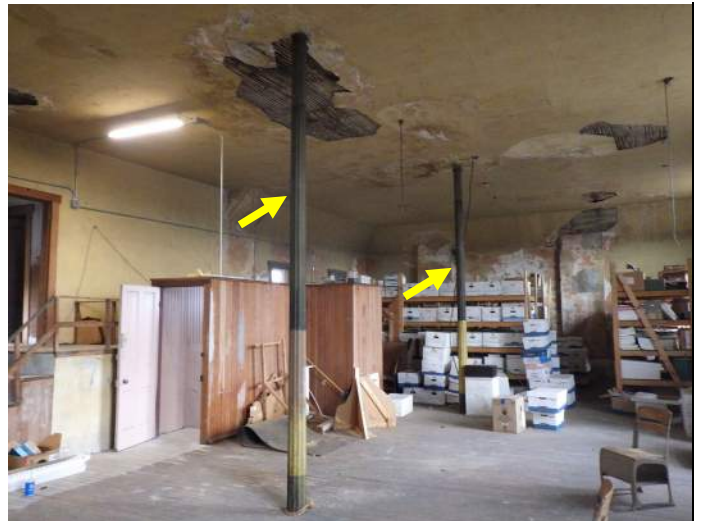
Steel columns supporting tower
