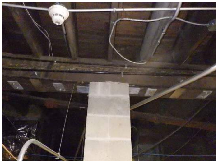
Reinforced timber beam and CMU pier
