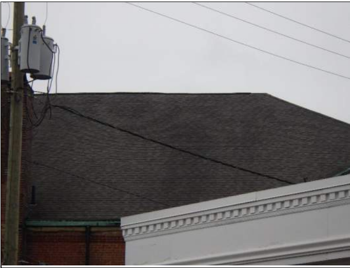
Overview of shingled roof
