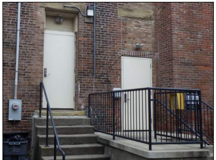
Typical metal doors
