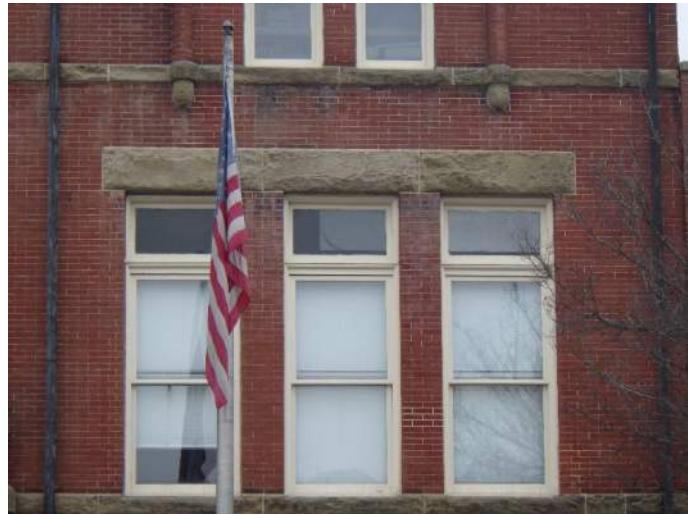
Typical vinyl windows
