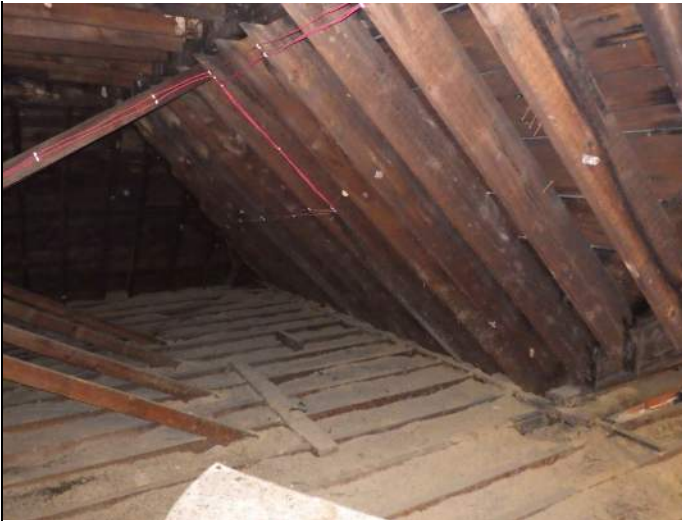
Overview of roof framing
