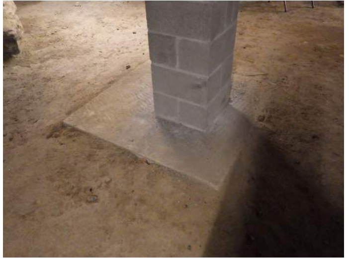
Water stains along valley rafter
