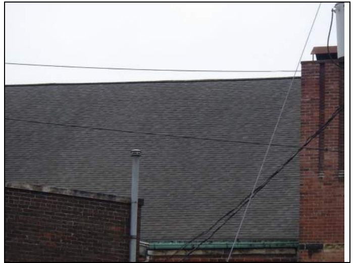
Overview of shingled roof
