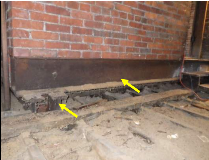
Steel beams below tower
