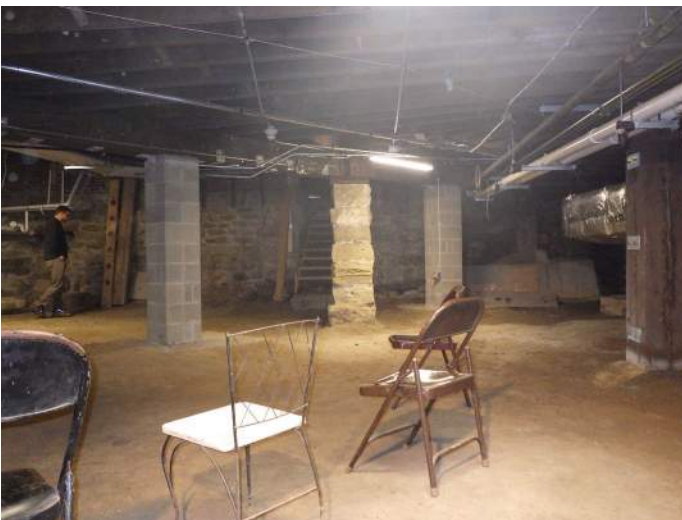
Overview of basement
