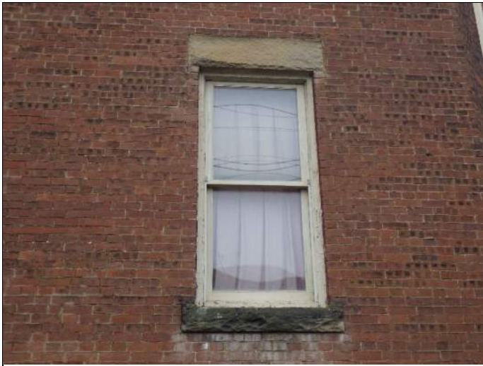
Typical wood-framed window
