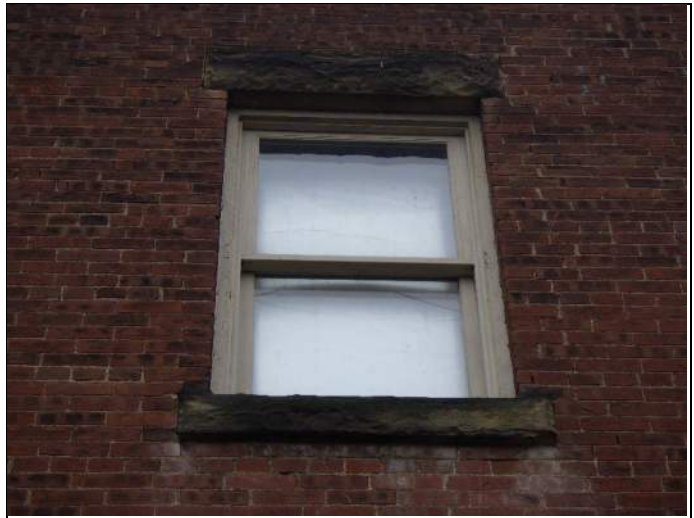
Typical wood-framed window
