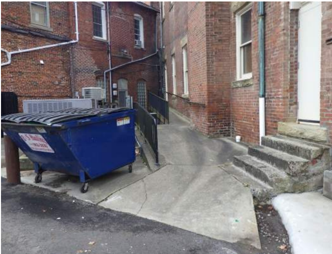
Accessible ramp in alley to auditorium
