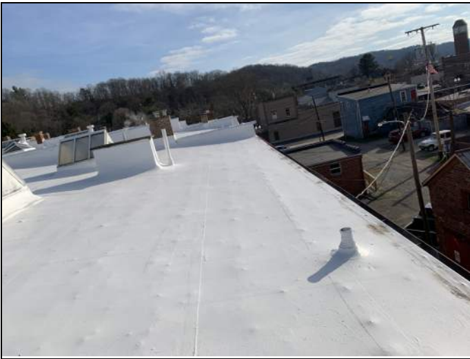
Gutter along south roof edge
