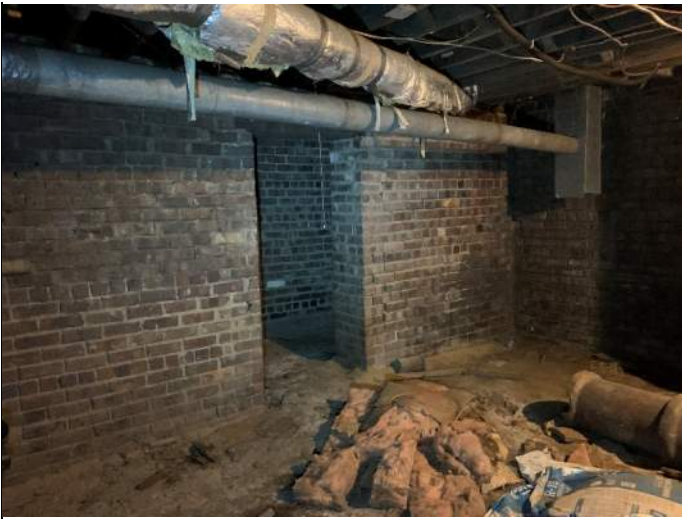
Typical brick masonry wall
