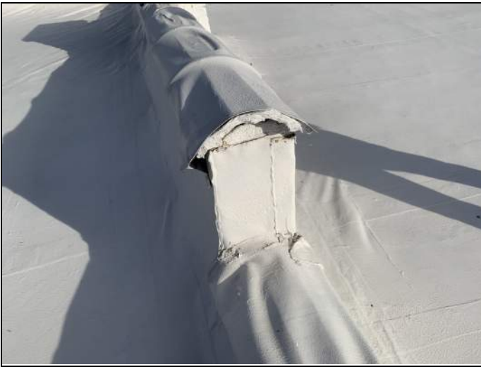
Open parapet end
