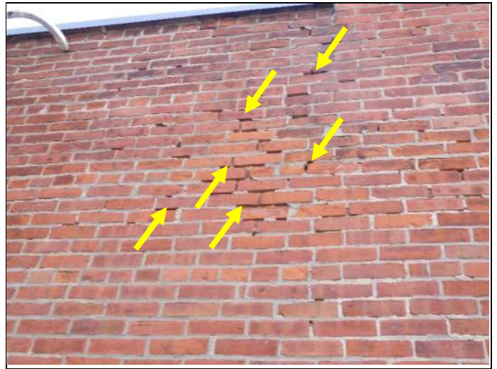
Mortar deterioration
