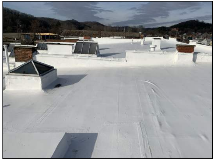
Overview of roof looking west
