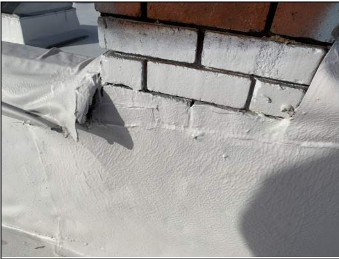
Membrane adhered to masonry
