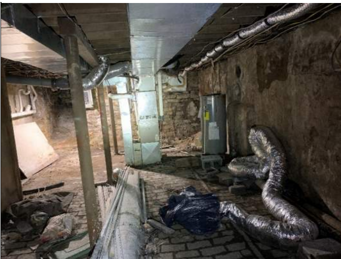
Typical brick floor
