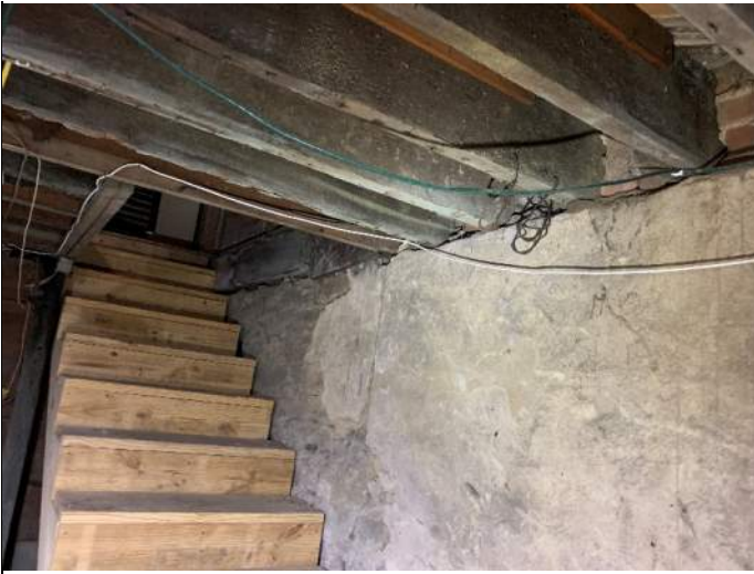
Typical stone masonry wall with plaster coating
