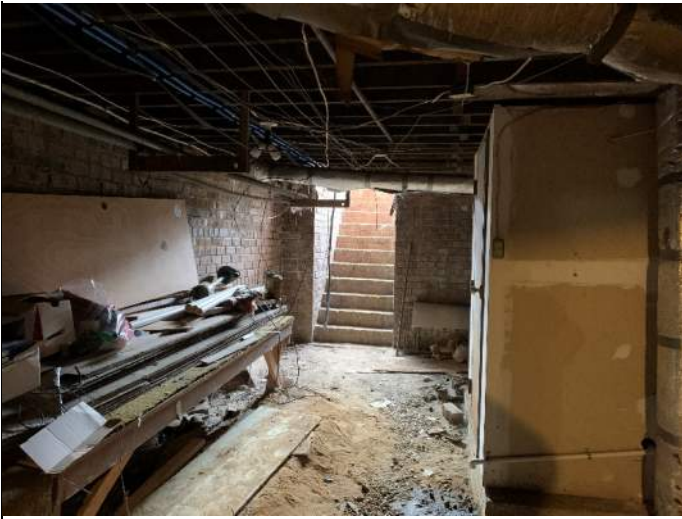
Typical "dirt" floor
