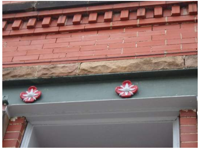
Typical stone and steel header above storefront
