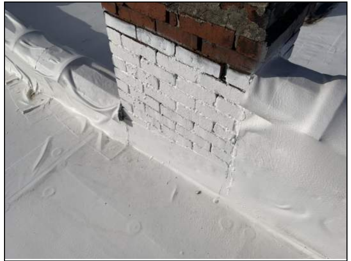
Membrane adhered to masonry
