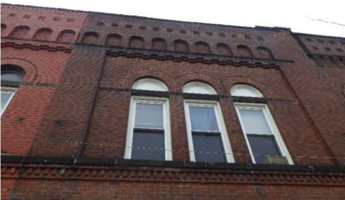
Typical vinyl framed windows
