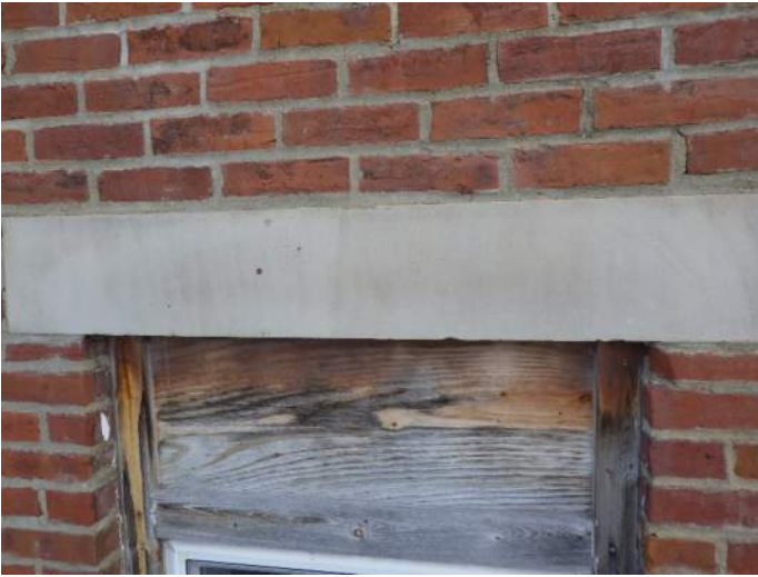
Typical stone lintel above window
