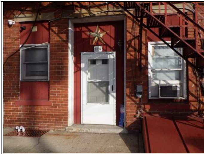
Typical first story rear entrance
