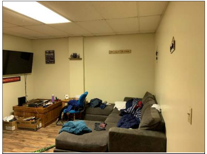
First-story residential space
