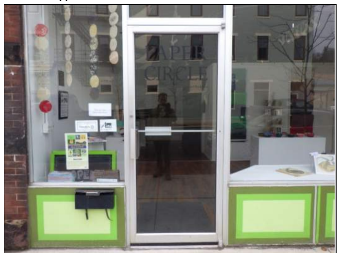
Typical aluminum framed door
