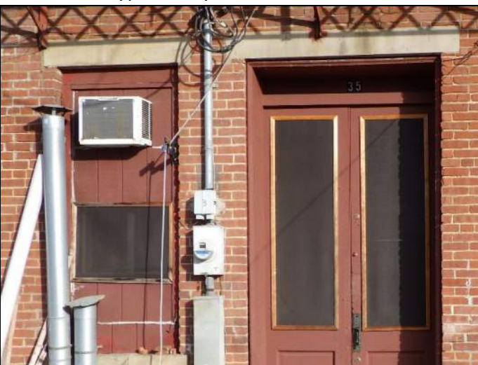
Typical wood framed windows and wood paneling
