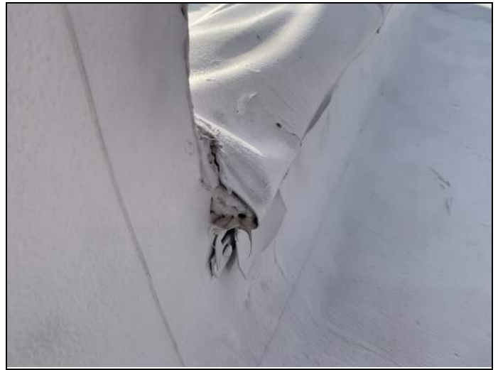
Open parapet end
