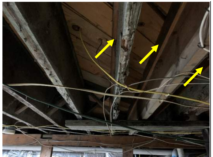
Floor joists "sistered" with new joists
