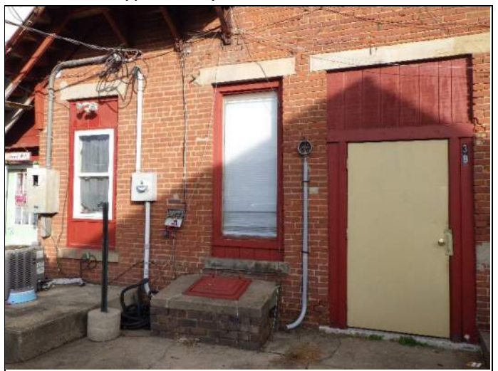
Typical wood paneling on rear elevation
