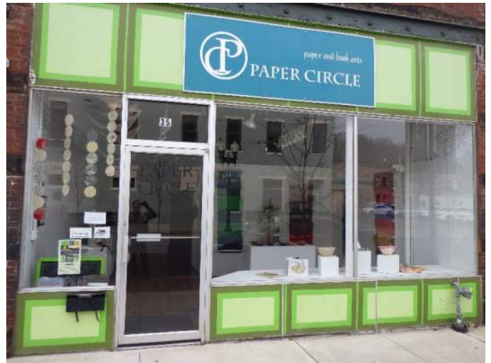
Typical anodized aluminum storefront
