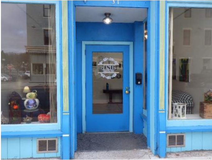
Typical wood framed door
