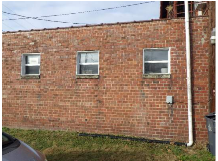
Typical vinyl framed windows
