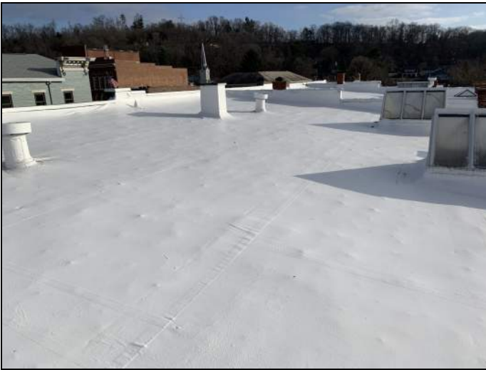
Overview of roof looking northeast
