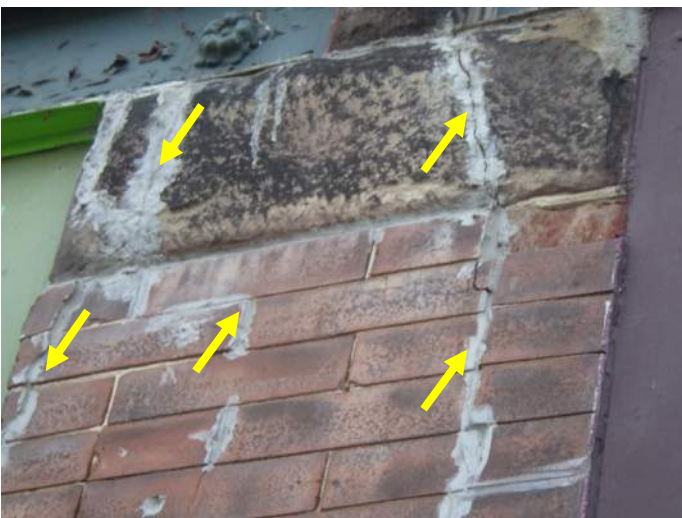
Previous stone and brick repairs
