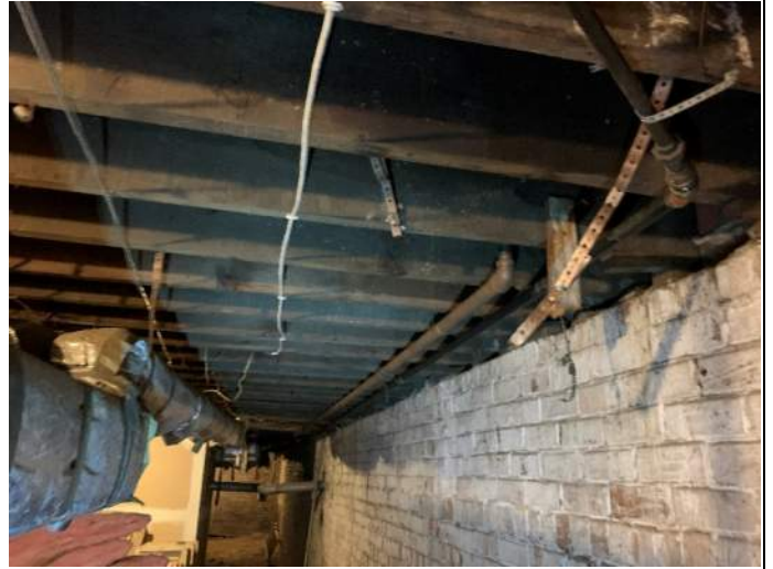
Typical floor joists supported by brick masonry
