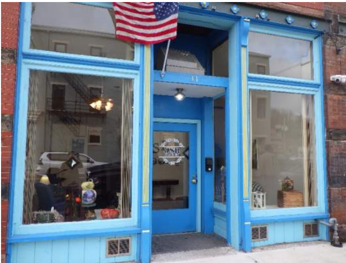
Typical wood-clad storefront
