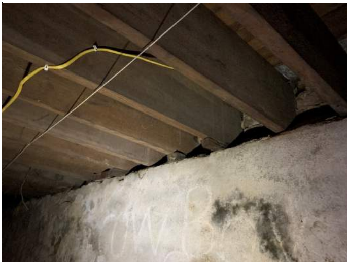
Typical floor joists supported by stone masonry
