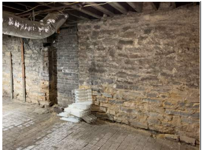
Typical star brick floor
