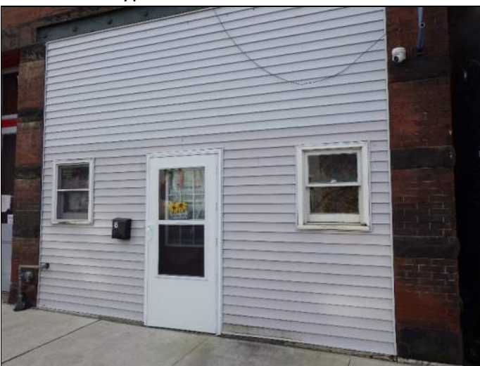
Typical vinyl-clad residential apartment
