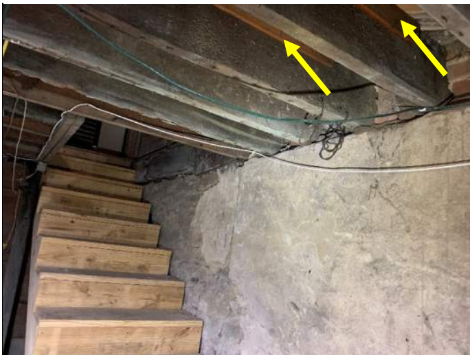
Floor joists "sistered" with new joists
