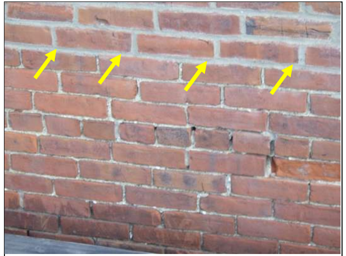
Typical cementitious mortar
