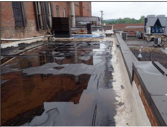
Large patch repair
