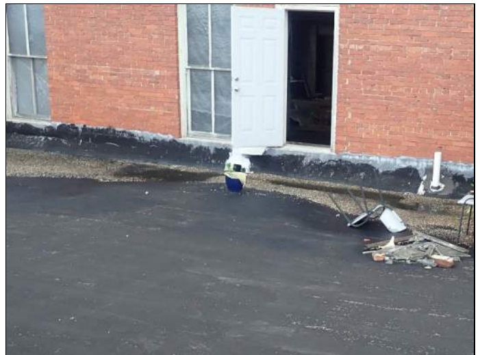
Single scupper at base of upper story wall
