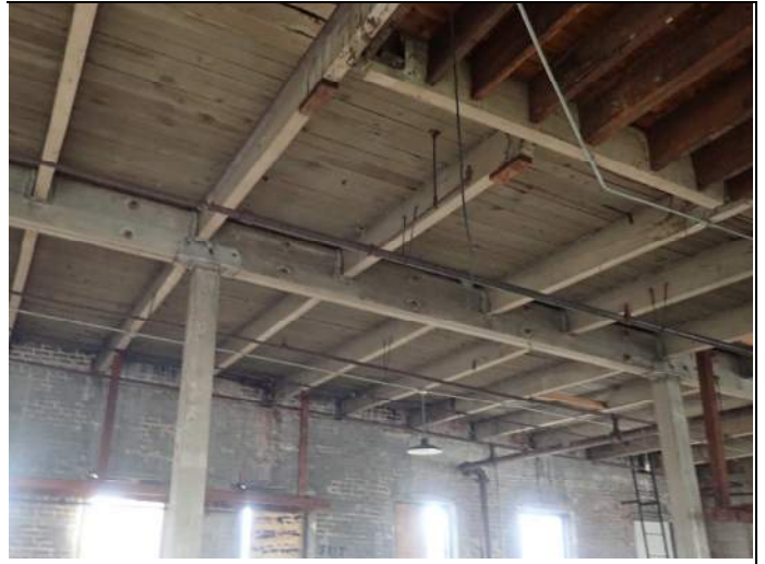
Typical framing of six-story building
