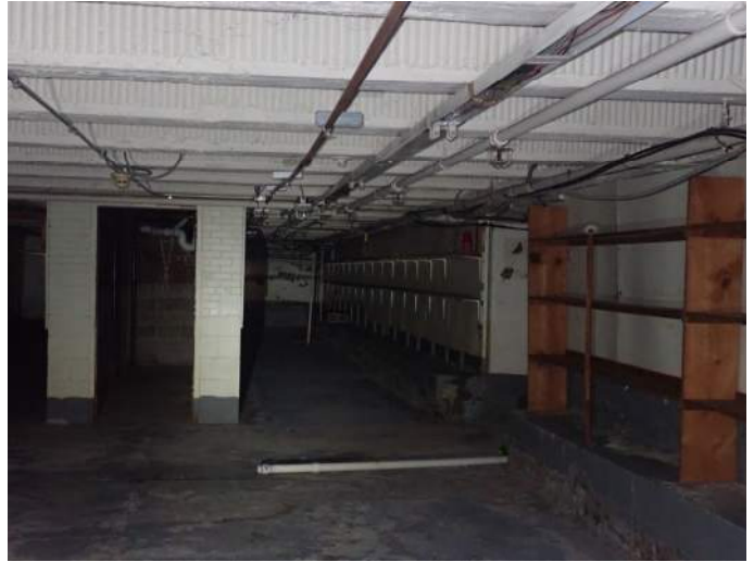
Overview of basement
