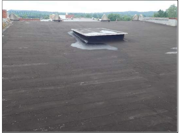
High roof side of middle roof
