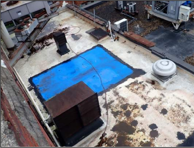
Overview of lower roof
