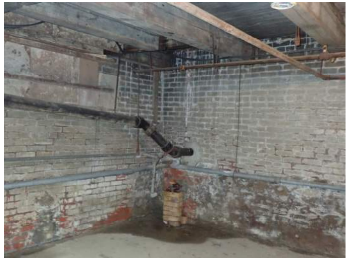
Overview of basement
