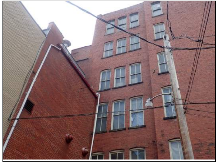
Partial north and west elevations
