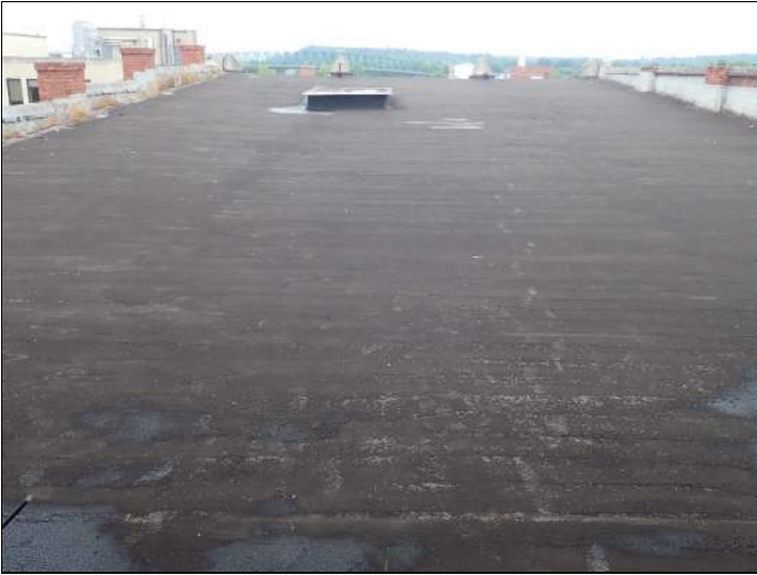
Overview of middle roof
