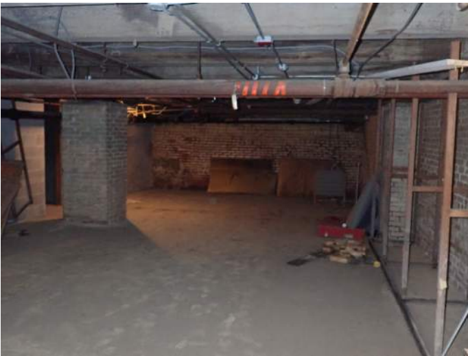
Overview of basement
