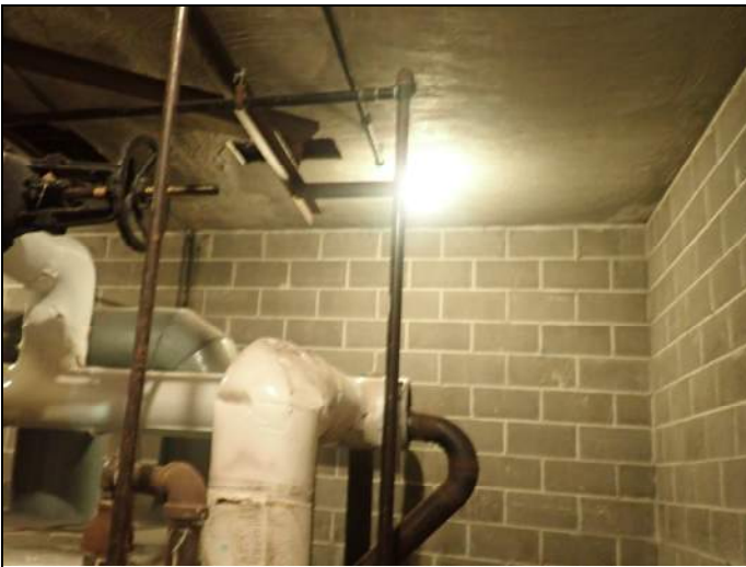
Overview of structure
