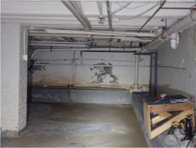
Overview of basement
