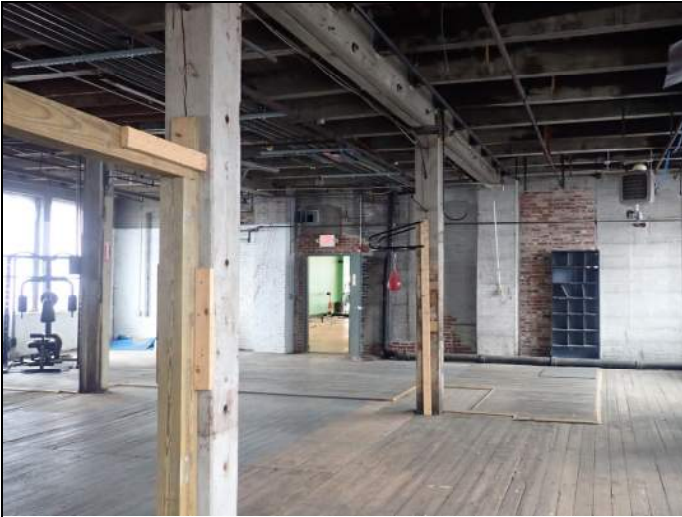
Typical framing of six-story building
