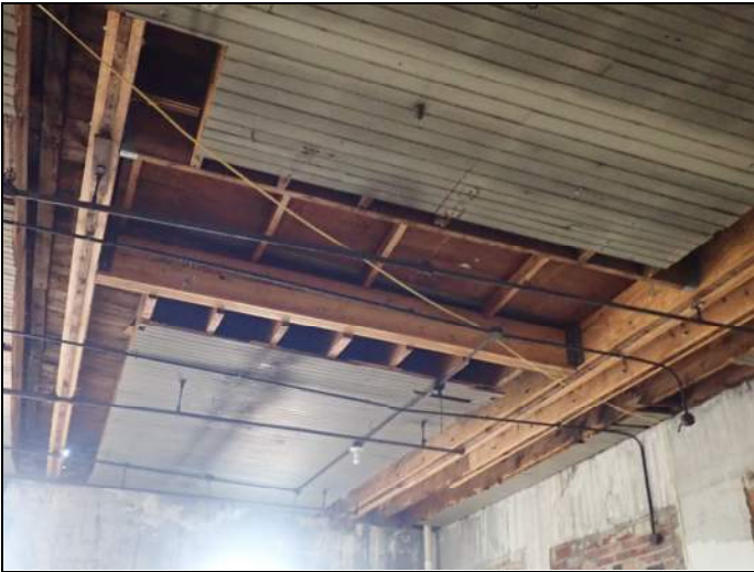
Prior structural repairs on roof
