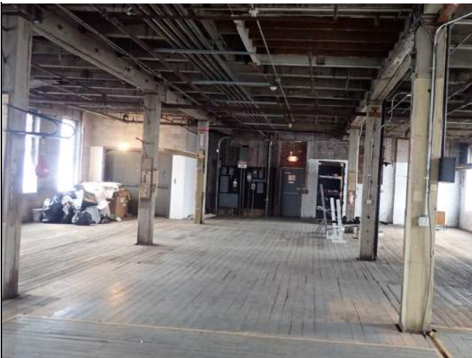
Typical framing of six-story building
