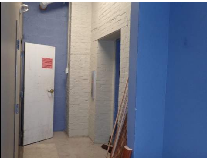
Main elevator at elevated first story
