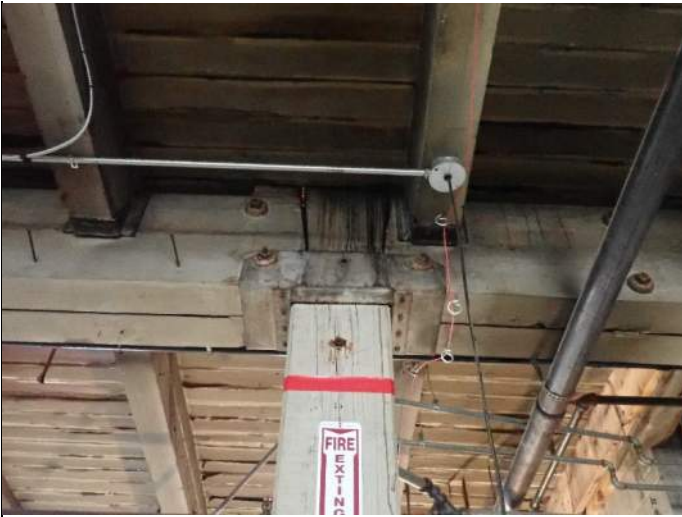
Typical beam and column connection
