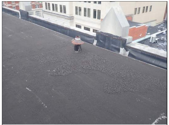
Typical condition of the middle roof
