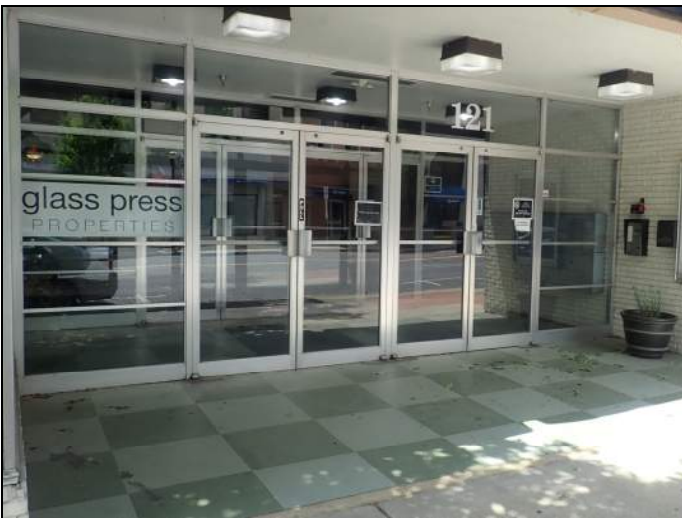
Anodized aluminum storefront system
