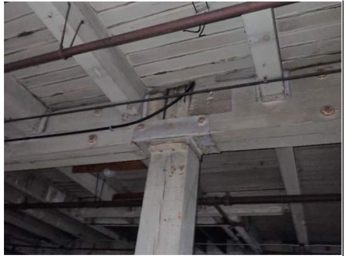
Typical beam and column connection
