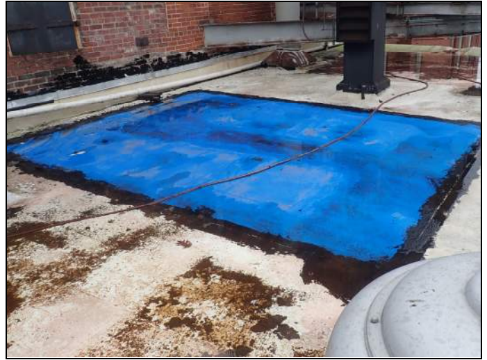
Large patch repair
