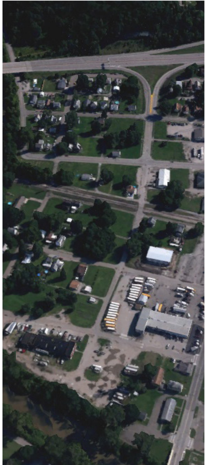
Above: Vacant and underutilized property is spread throughout the neighborhood, surrounded by commercial and industrial zoning districts.
